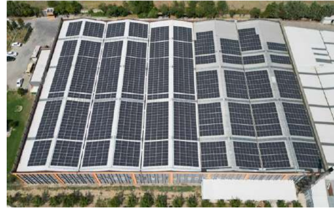
Cargill Balıkesir 2.735 kWp/ 2.400 kWe
